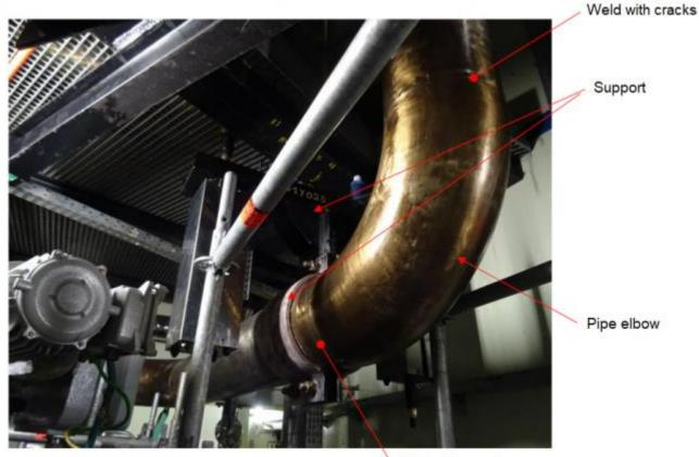
Weld with cracks
